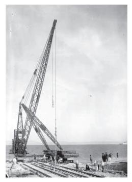
Photo 4. The construction of the seaport of Gdynia – a crane being operated during the construction of the port of Gdynia (Source: National Digital Archives)
