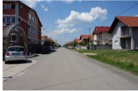
Fig. 16. Busije street with a school building. Morovićkih šuma street. Author: Magdalena Reškć (June 2022).
