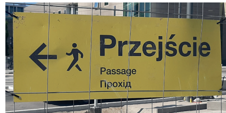
Figure 9. Organisational / informational sign at a construction site
