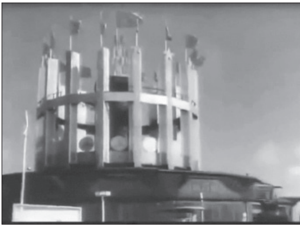
Il. 1. Polska Kronika Filmowa : reverse modeling – USSR Pavilion at the Poznań International Fair (source: PKF 18/49, still)
