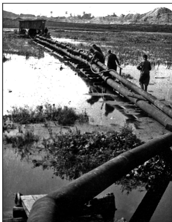
Fig. 3. Drying of the ground surface in the area of the future Niesłusz opencast (photograph from DMK archives).
