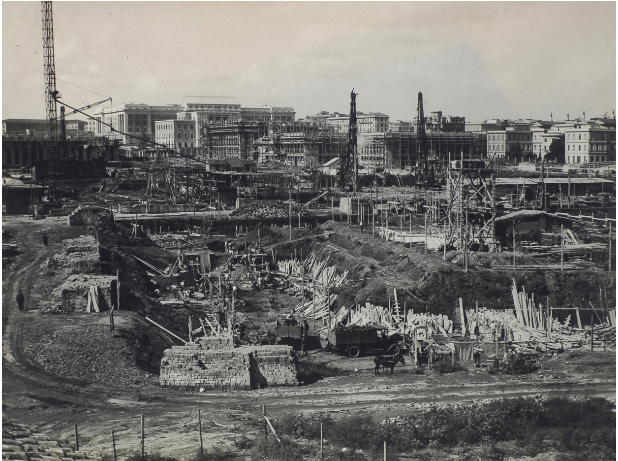
Fig. 6. Excavations for the foundations of the Sapienza Campus buildings, July 1933. (Author: unknown. Source: Sapienza Historical Archive).
