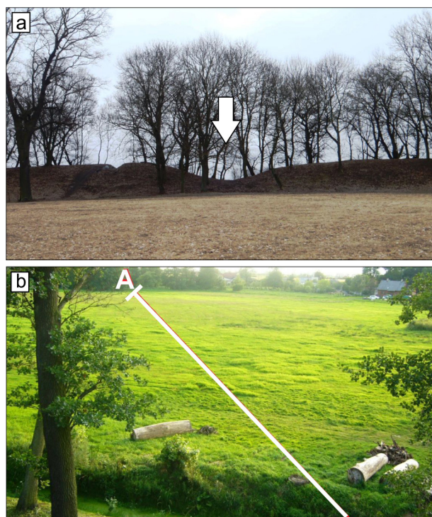
Fig. 4. View of the stronghold. a) lowering in the embankments, b) view to the west of the stronghold with marked cross-section line A-A' exceeding the boundary of the embankments.
