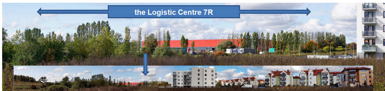
Fig. 11. Buildings of the Logistic Centre 7R Gdańsk Kowale. View from Zeusa Street. Photo by J. Poczobut, 2019.
