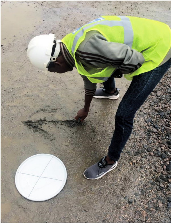
Fig. 3. Ground Control Point (GCP) station selection and marking.
