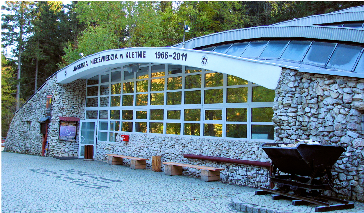
Fig. 4. Entrance pavilion of Bear Cave (photo A.Marek 2021).
