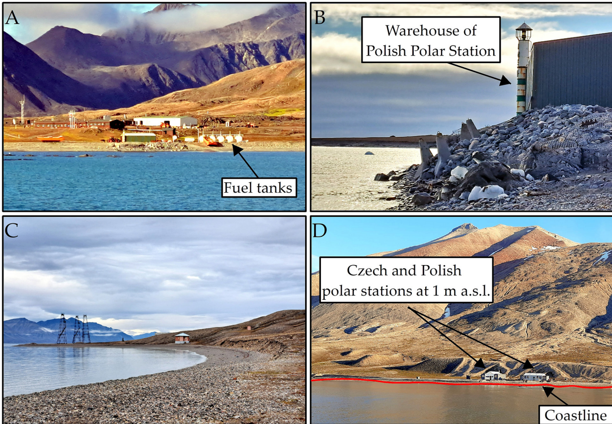
Fig. 7. Examples of coastal buildings and facilities in Svalbard vulnerable to damage due to their location: A - The Polish Polar Station buildings and facilities on the northern, eroding coast of Hornsund; B - The warehouse of the Polish Polar Station, as a result of long-term erosion of the Hornsund coast, is now on the edge of the land. Its southern wall has already been reinforced several times to prevent damage to the building; C - The remnants of 20th century mining activities are still visible in the landscape of Spitsbergen; D - Polish and Czech polar station buildings located ca. 25–30 m from the coastline at the bottom of Pyramiden Hill. The photo was taken from Petuniabukta Bay. Photo by Z.Owczarek (A, B, C), O.Kostrzewa (D).
