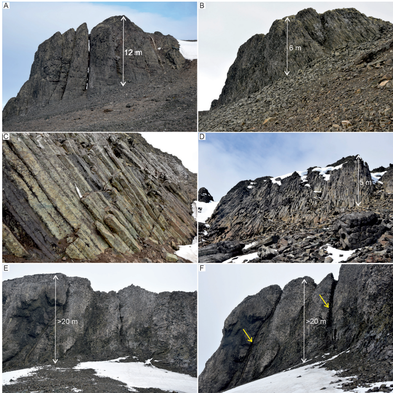
Fig. 3. Different arrangements of columnar jointing in andesites of the Jersak Hills. A – narrowly-spaced vertical joints, with additional master joints spaced 1–3 m apart (cliffs are 12 m high); B – inclined columns dipping into the slope; C – inclined columns concordant with the slope (Schmidt hammer for scale); D – transition from vertical (right) to inclined columns (left); E – flat-lying columns exposed in a high cliff; F – vertical zones of hydrothermal alteration (marked by arrows).
