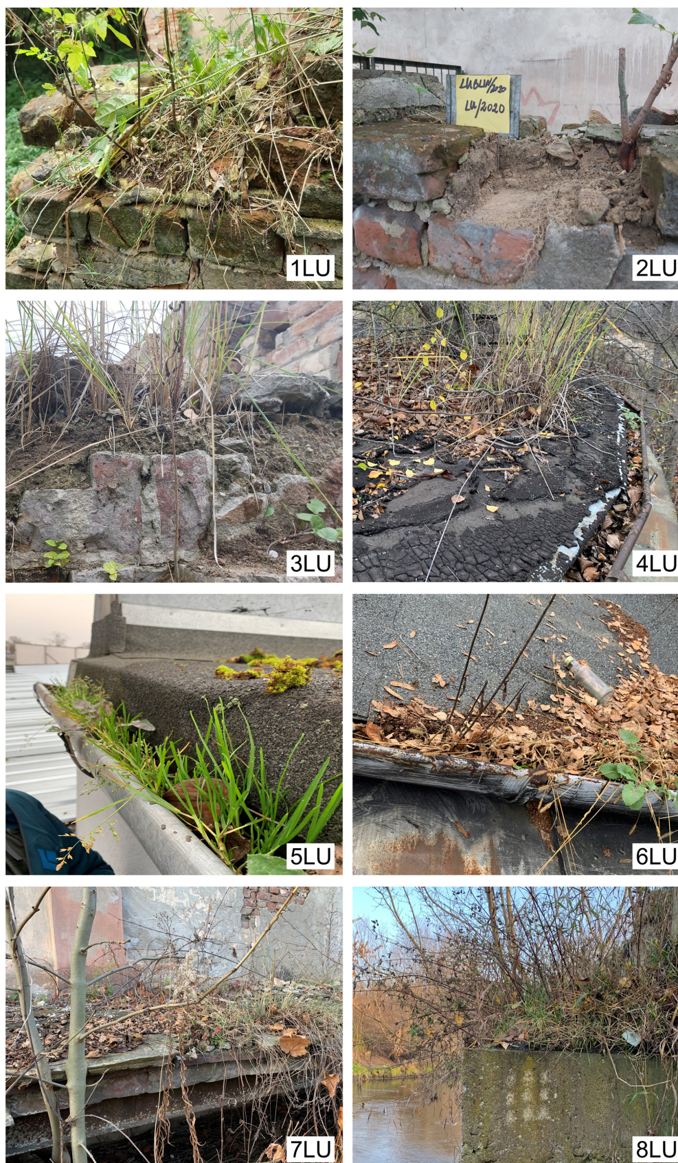
Fig. 2. Analysed soils: 1LU - watermill, 2LU - brick wall, 3LU - industrial plant (dyehouse), 4LU - railway outbuilding, 5LU - industrial plant, 6LU - car garage, 7LU - railway ramp, 8LU - concrete bridge pillar.
