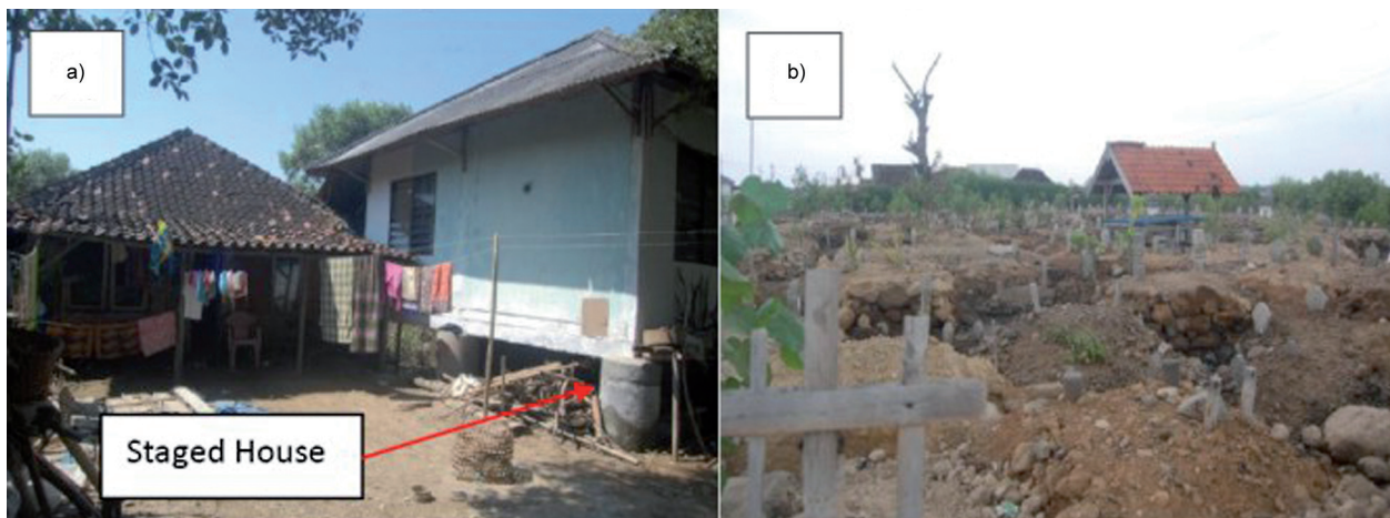
Fig. 8. (a) Staged house built by Tambaksari inhabitants, (b) elevated ground level to maintain the cemetery.
