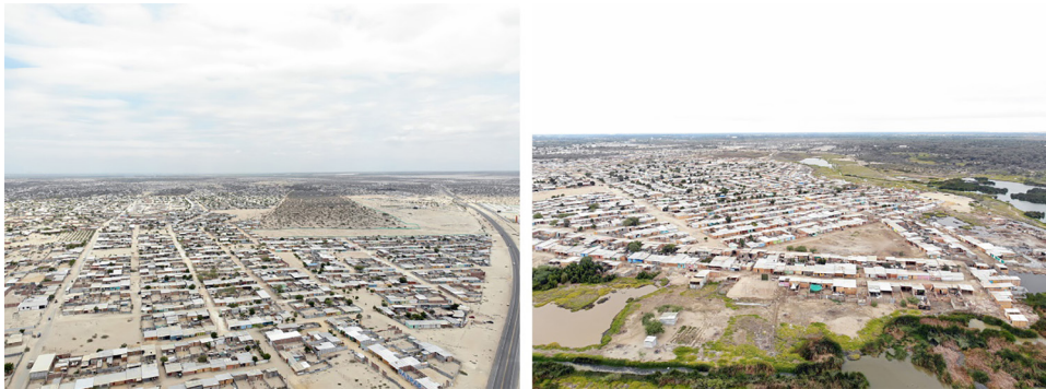
Fig. 2. Photographs 2022. Left: Informal urban expansion of the last two years without access to basic services. Right: Settlement close to natural wetlands vulnerable to flooding
