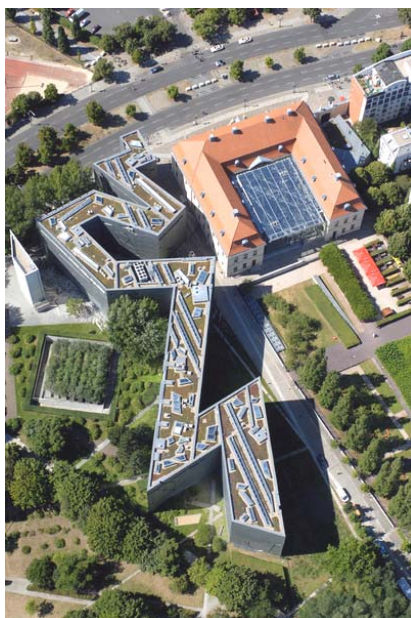
Fig. 1. Daniel Libeskind's Jewish Museum in Berlin. Bird's eye view [online]. E-architect [access: 2014-02-14]. Available at: < http://www.e-architect.co.uk/images/jpgs/berlin/juedisches_museum_cguenterschneider_3.jpg >
