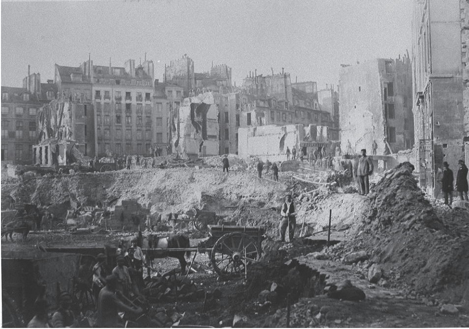
Figure 7. Works during the construction of avenue de l'Opéra, at Butte du Moulin and rue Saint-Roch. Photo Charles Marville, 1862
