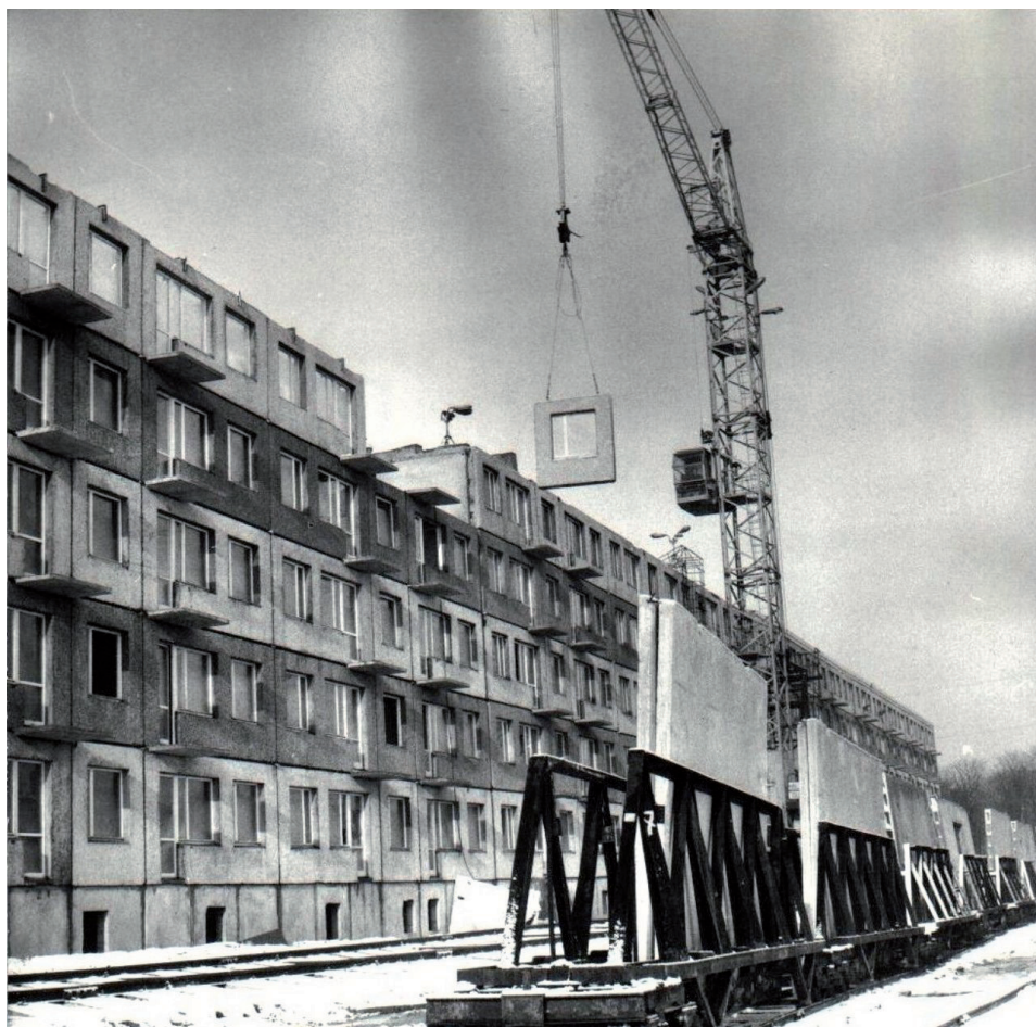
Figure 3. Construction of the Wichrowe Wzgórze estate in Poznań, 1976. At the time, the Soviet Land Estate was under construction. Author of the photo: Henryk Kamza
