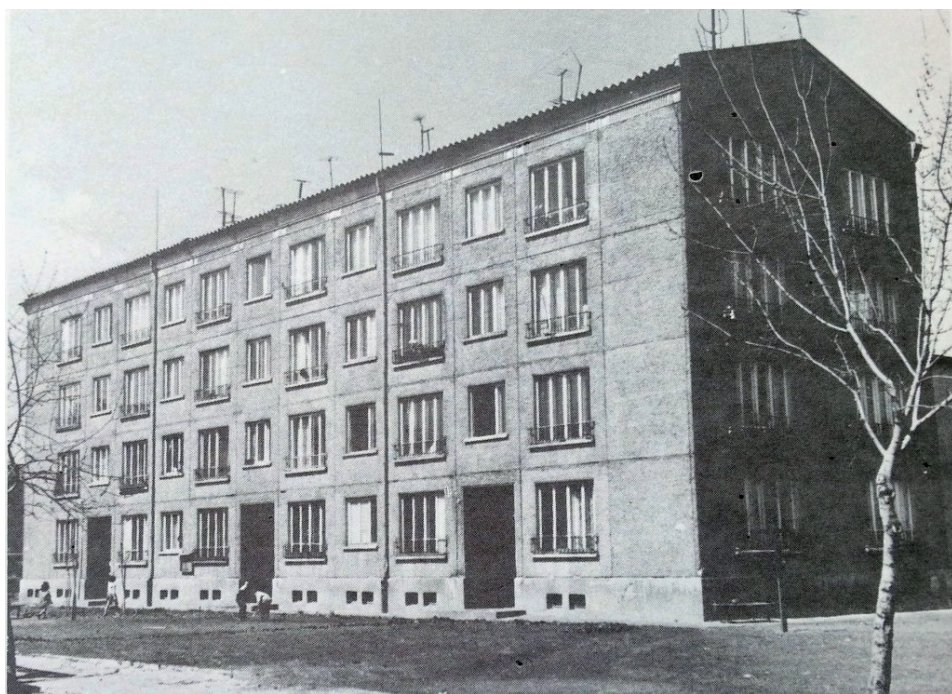
Figure 1. The first panel block in Bulgaria (built in Sofia in 1958)
